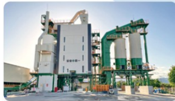
Asphalt plant (AP-Related Business)
