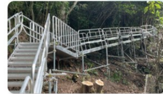
Temporary construction equipment (Other Business)
