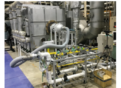
Hydrogen burners (in development)
