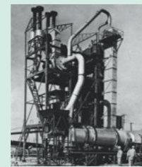
1958: Nikko's first asphalt plant completed
