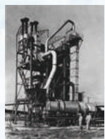
Nikko's first asphalt plant produced (1958)
