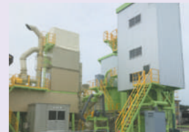
A plaster-based solidification material manufacturing facility A plant facility which manufactures gypsum hemihydrate from dried gypsum powder, which is blended with cement and lime to manufacture solidification material.
