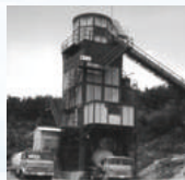
Development of u-type concrete plants (1977)
