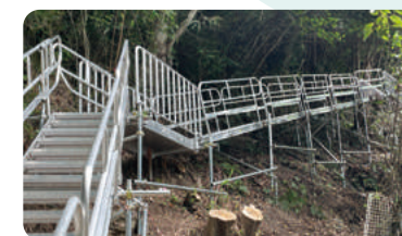
Temporary construction equipment (Other Business)
