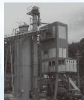
Development of compact concrete plants (1979)
